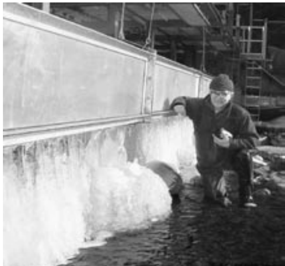
An unusual freezing period and associated low stream flows at Auke Creek weir in March 2006 resulted in the massive accumulation of ice on the fish counting weir. Ice was removed daily to keep the weir operational.
