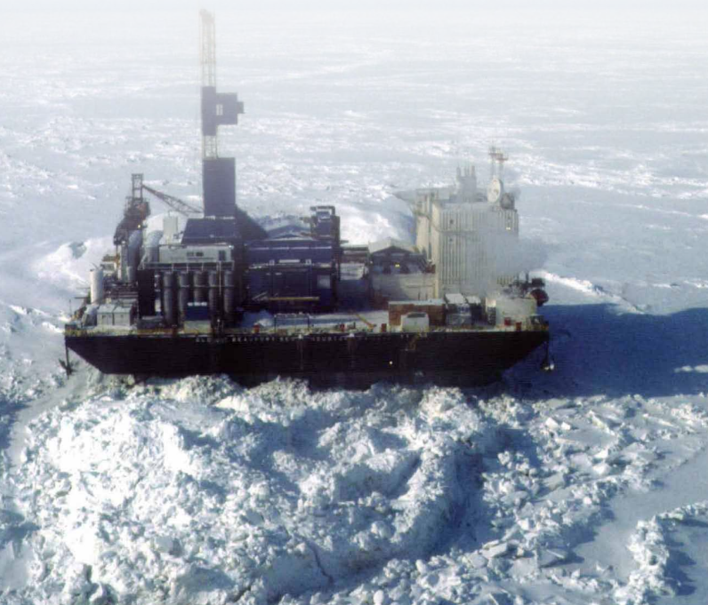
Concrete island drilling system in sea ice. Photo: Dept. of the Interior.
